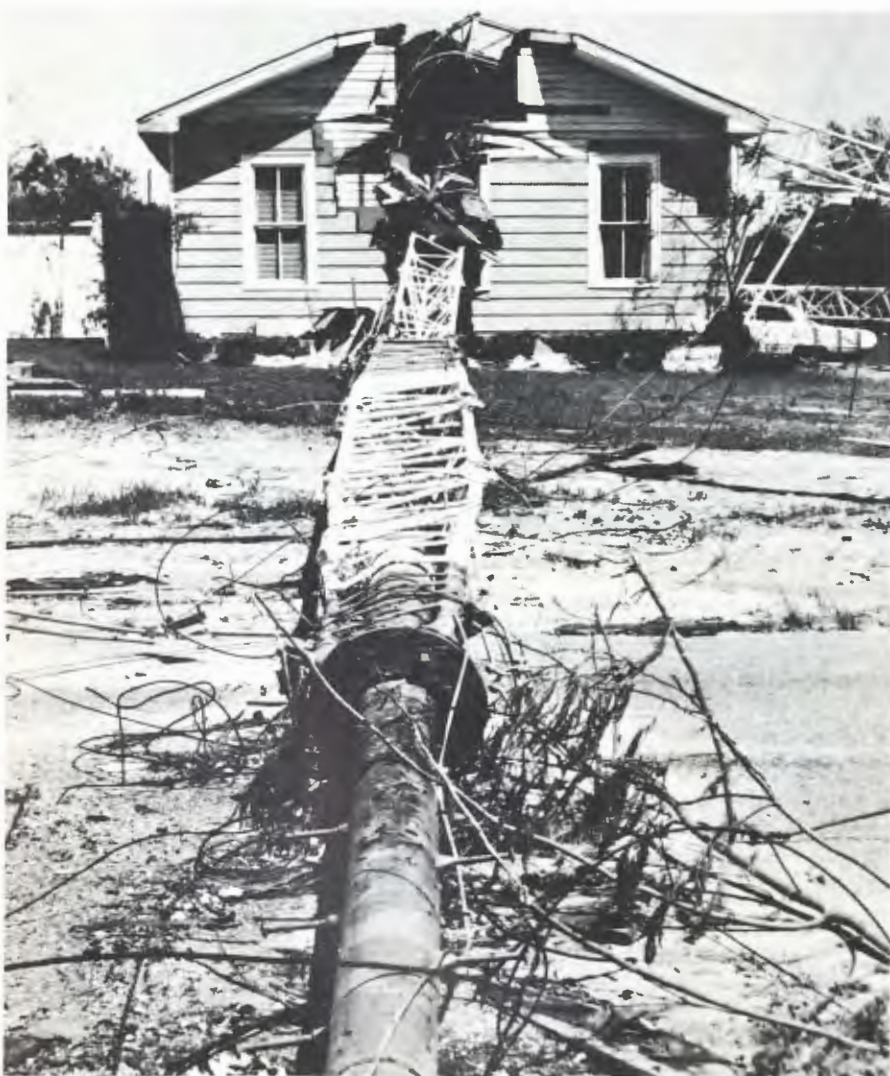
Fig. 1 Shown here is the WGCM tower after it toppled into one of the station buildings. BE will continue its coverage of emergency broadcasting in the November issue.
